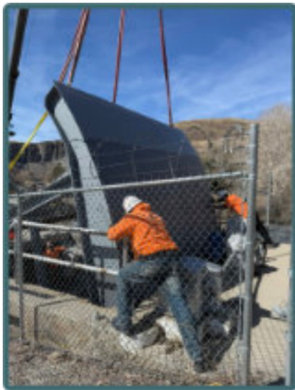
Crews place the refurbished radial gate.
