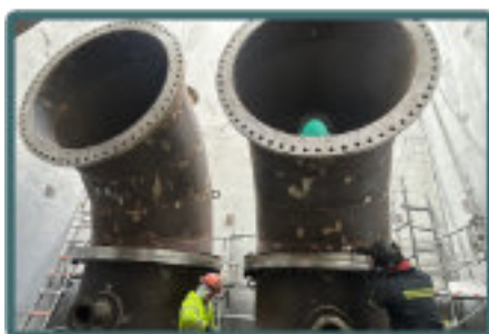
Installation of new 90-degree elbows for the bypass pipe.
