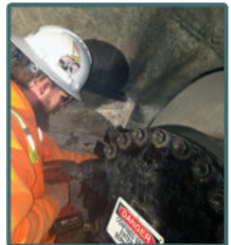
Removing manway on DC Penstock
