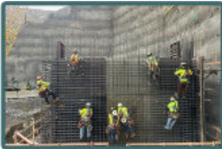
Construction crew installing wall reinforcement for Level 2.
