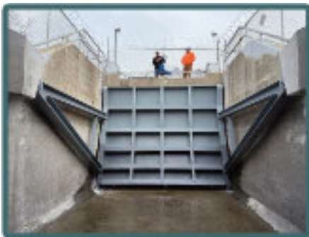
Inspection of refurbished radial gate.
