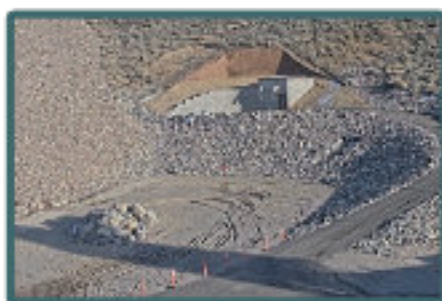
Riprap placed around the tie-in vault (construction camera, September 2, 2025).
