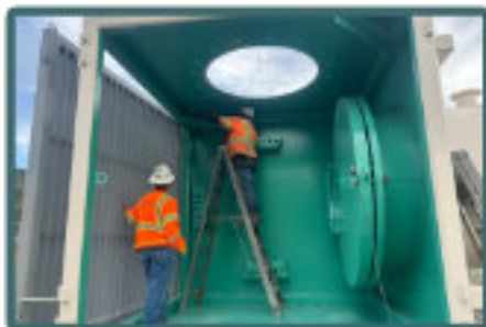
New 72-inch bypass trash rack.
