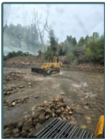
Weber-Provo Diversion Forebay Cleaning
