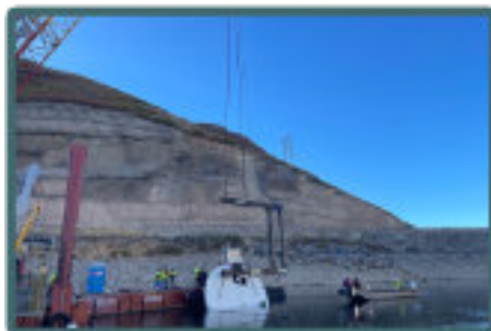
192-inch bulkhead positioned near vertical, ready for installation.
