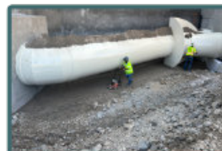
Compaction of bedding sand beneath the 72-inch bypass pipe.
