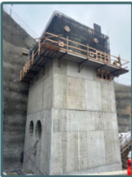
Rebar and block-out forms completed for Level 4 walls.
