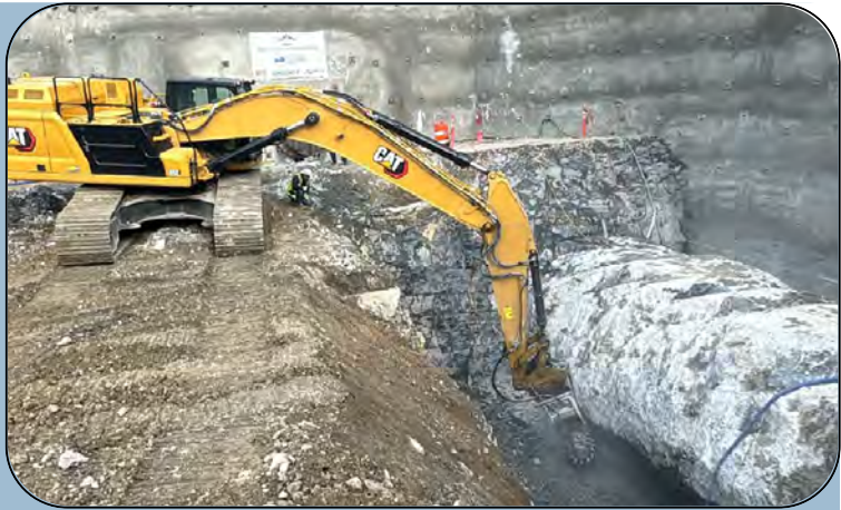
Uncovering Concrete Penstock Tunnel
