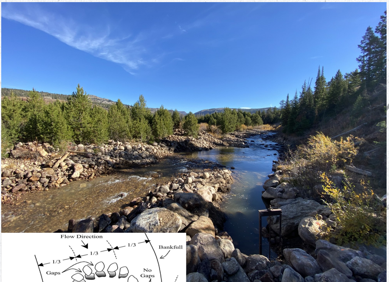
J-hook cross vane in the upper Provo River
