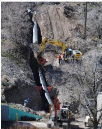
ULDC North Branch Pipeline
